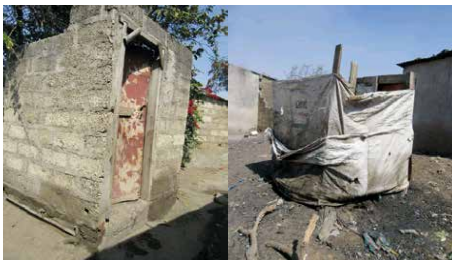
Figure 1: Types of pit latrines being used in low income areas of Lusaka
