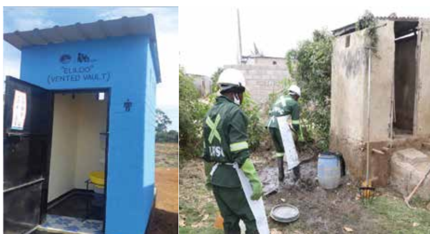
Figure 2: Improved toilet constructed in George compound and safe pit emptying service provision by contracted service providers.
