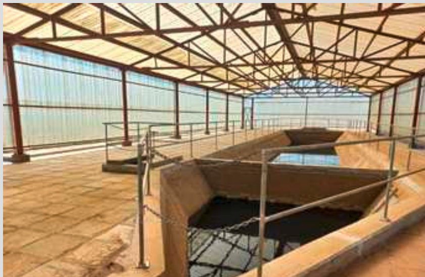
Newly Constructed Faecal Sludge Treatment Plant at Matero, Lusaka Province, NWASCO 2022
